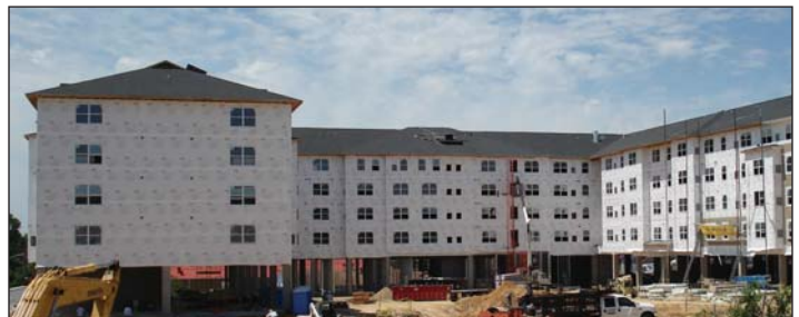
Ashbury Courts Concrete and Wood Frame
